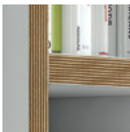
Plywood edges detail
